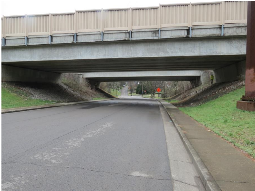
CLEARANCE VIEW LT. SIDE
