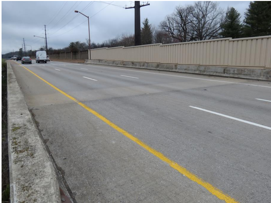
VIEW ACROSS TOP OF WEARING SURFACE WBL
