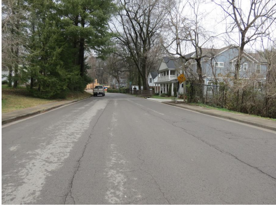
VIEW LOOKING NORTH ON CRAIG AVE.
