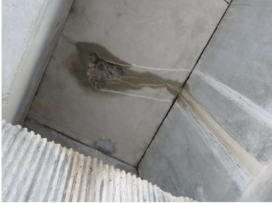
DECK PANEL BAY "D" ABUT. #1 OVERALL VIEW
